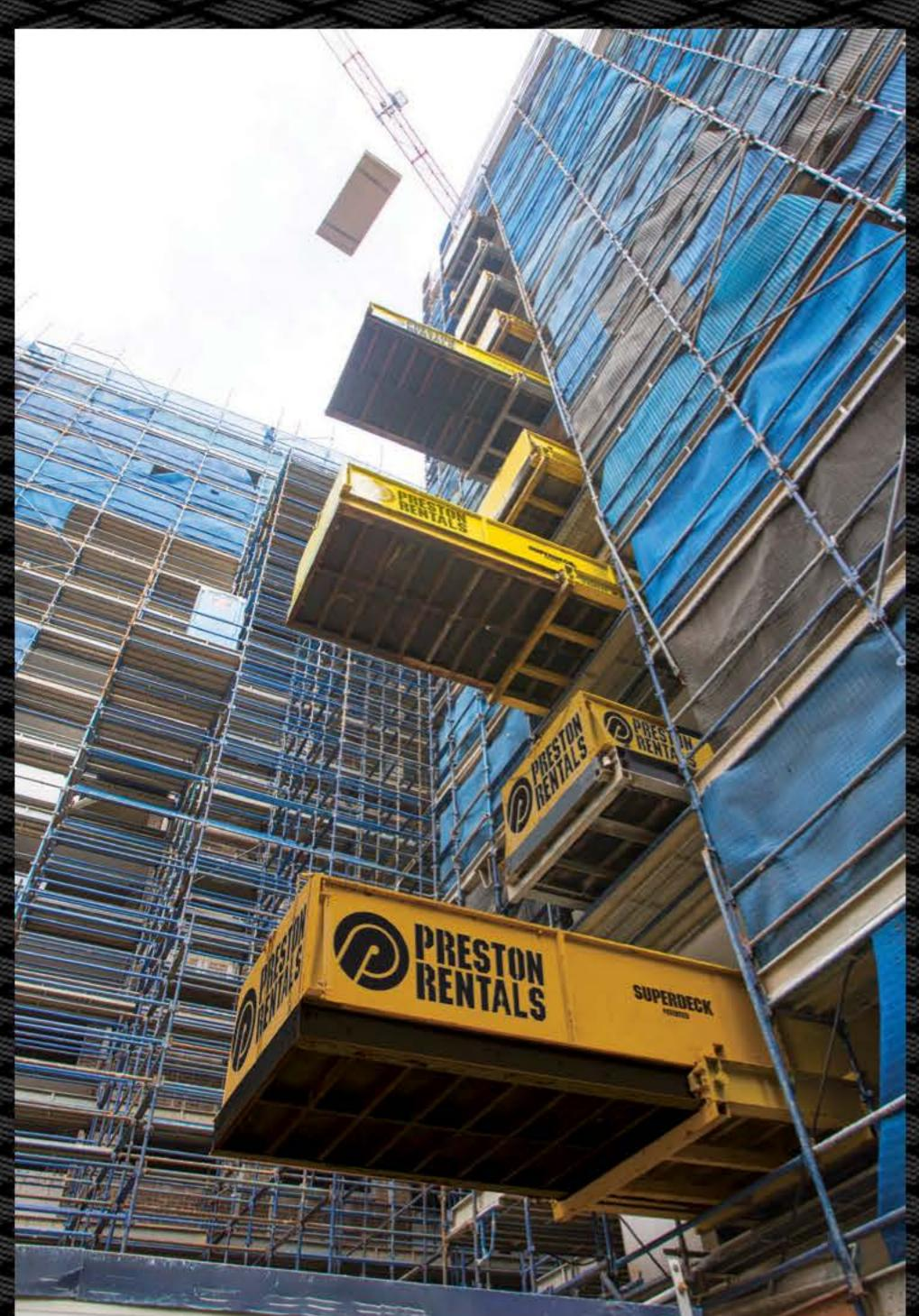
The ® PRESTON RENTALS Superdeck® Retractable Loading Platform System is ideally positioned vertically, one above the other, for fast delivery of building materials by a crane.
