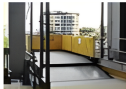
Loading Platforms Ramp
